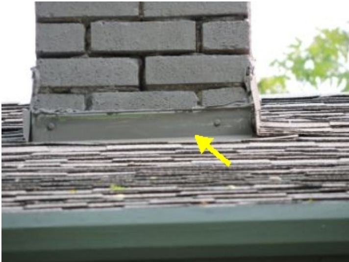
Example view - flashing at chimney
