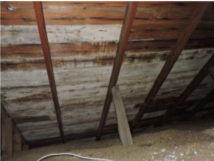
Example view - attic structure
