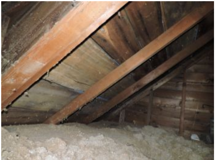
Example view - attic structure
