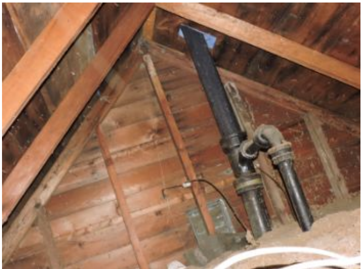
General attic view - plumbing stack
