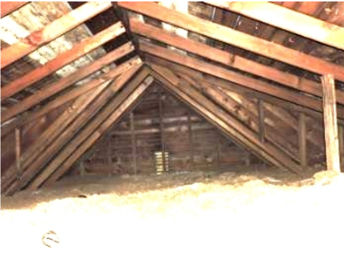
General attic view - west
